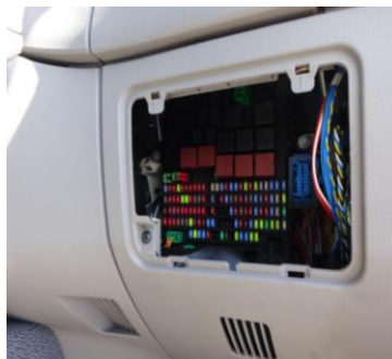
Figure 7-2.2 Inside View - Electrical Junction Box Location
